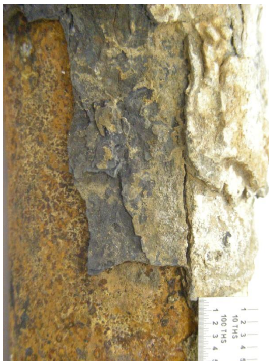
Figure 5. Thick OD deposit and severe wastage, refuse fired SH tube.
